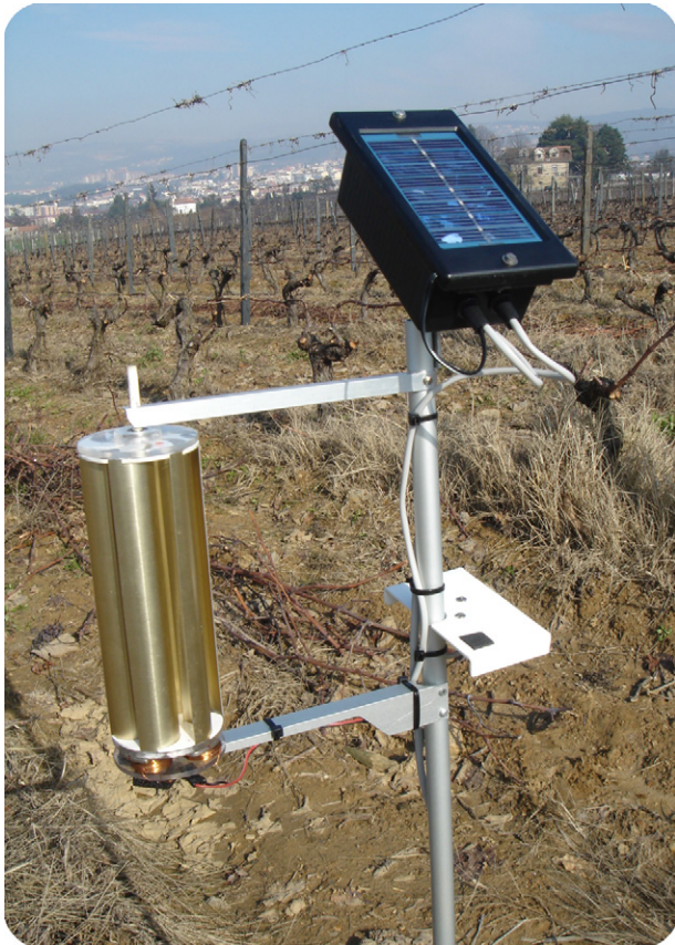
Fig. 11 – Experimental evaluation of the WDAP in a vineyard management zone. In this setup, the energy was supplied by the sun, wind and sporadically by irrigation water.
