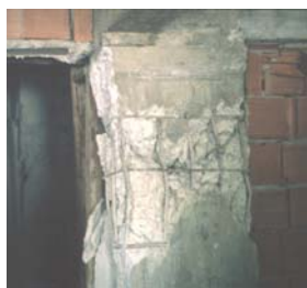
Figure 2.31 - Column shear failure (Aschheim, 2001)
