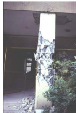
Figure 2.29 - Shear and bond failure at the mid-height of a RC column during the 1985 Mexico city earthquake (EASY, 1997)
