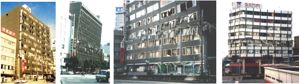
Figure 2.18 - RC frame structures with a mid-height collapse (EQE, 1995; KOBEnet, 1995)
