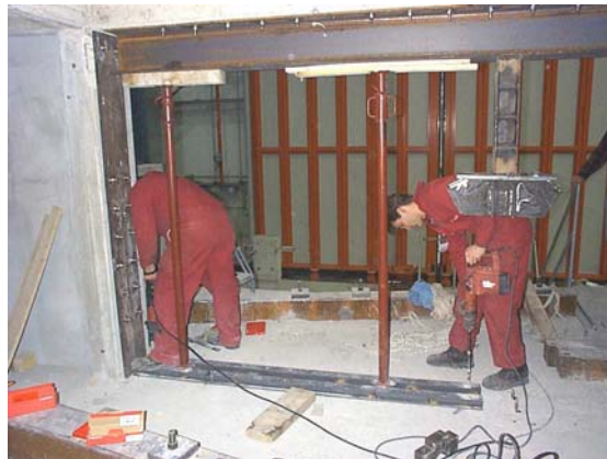
Figure A.48 - Bottom-beams: drilling
