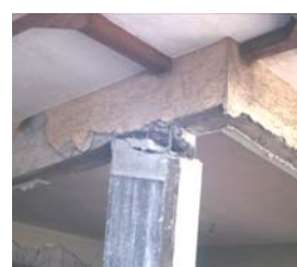
Figure 2.27 - Bar pullout-columns (Aschheim, 2001)
