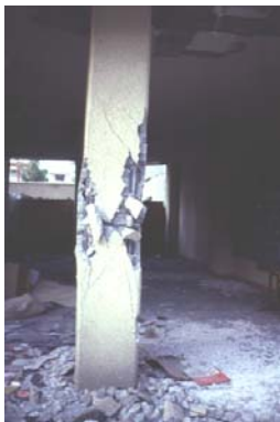
Figure 2.29 - Shear and bond failure at the mid-height of a RC column during the 1985 Mexico city earthquake (EASY, 1997)
