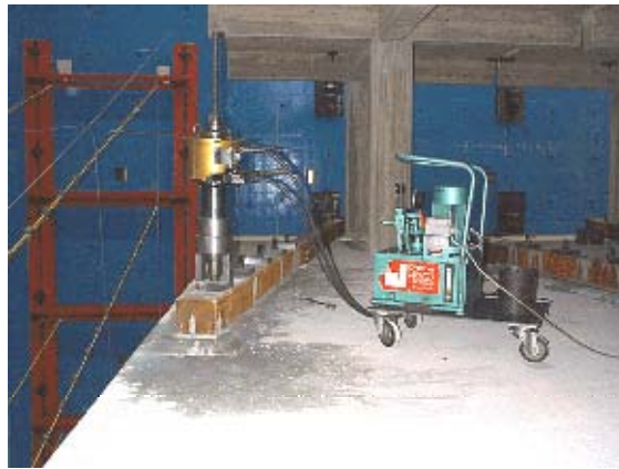
Figure A.14 - Vertical connectors pre-stressing (to attach the actuators at the steel load frame)
