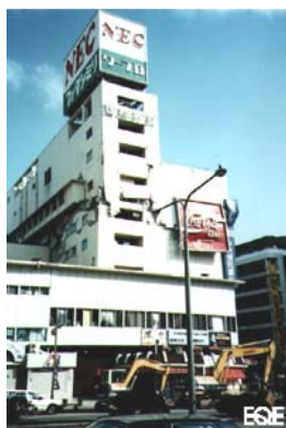
Figure 2.20 - Badly damaged irregular RC building in Sannomiya (EQE, 1995)
