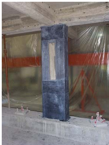
Figure A.56 - Column repaired with carbon fibre materials
