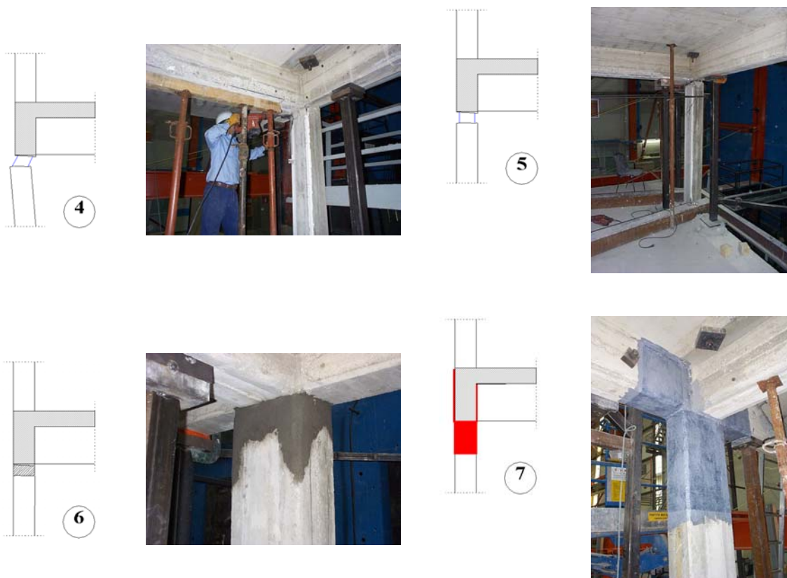
Figure A.52 - Repair operations (steps): 4 – remove concrete at the top of the damaged column; 5 – relocation of the column; 6 – concreting of the column/joint; 7 – strengthening with carbon fibre
