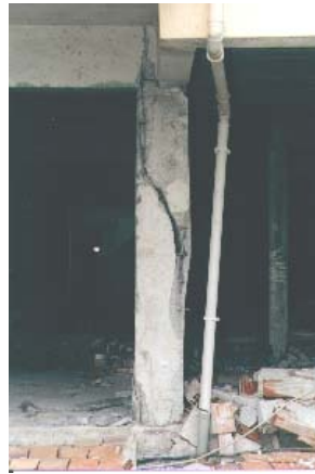
Figure 2.28 - Column shear failure examples: a) 1979 Montenegro earthquake (EASY, 1997); b) 1999 Izmit earthquake (note the to lack of transverse reinforcement - Saatcioglu et al. , 1999)
