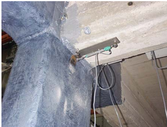
Figure A.32 - Instrumentation in repaired external joints (relative displacement transducer)
