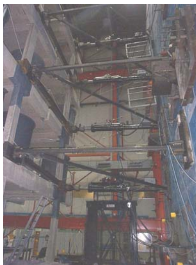
Figure A.16 - Fixings to the reaction-wall, steel pined bars connecting the two frames and actuators
