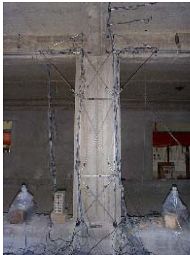
Figure A.21 - Instrumentation: strong-column at 1 st storey
