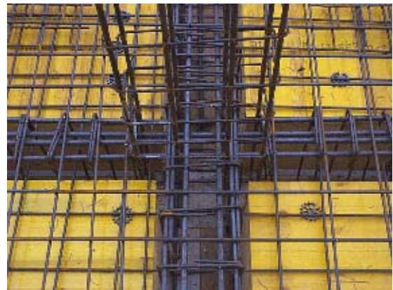
Figure A.6 - Joint detail
