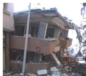
Figure 2.27 - Bar pullout-columns (Aschheim, 2001)
