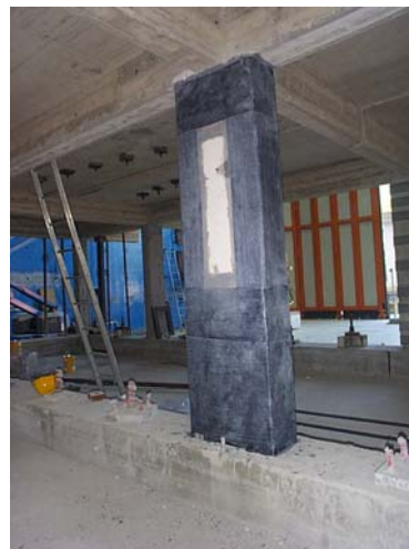
Figure A.56 - Column repaired with carbon fibre materials
