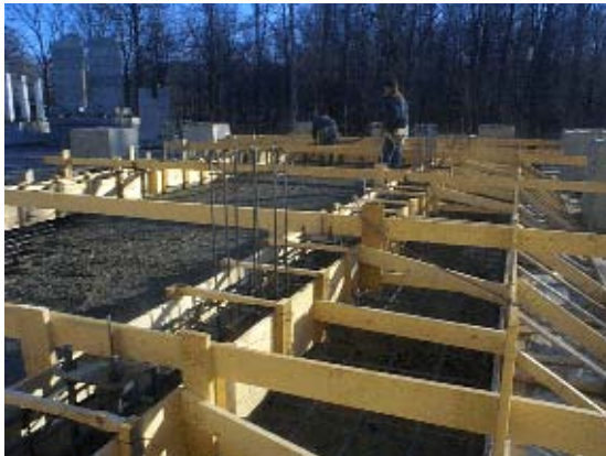
Figure A.3 - General view of the base foundation (concrete casting)
