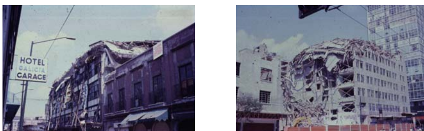
Figure 2.42 - Building failure due to the higher modes effect during the 1985 Mexico city earthquake (EASY, 1997)
