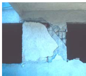
Figure 2.31 - Column shear failure (Aschheim, 2001)
