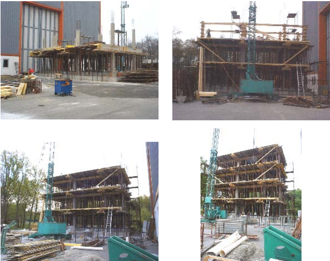
Figure A.10 - Construction at various phases (general views)
