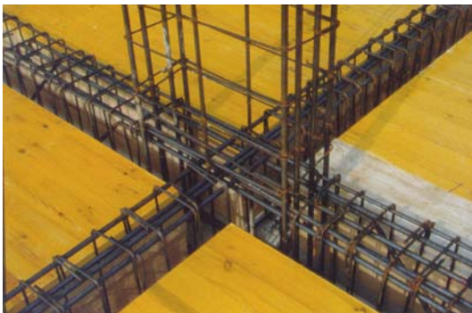
Figure A.9 - Joints and columns reinforcement details
