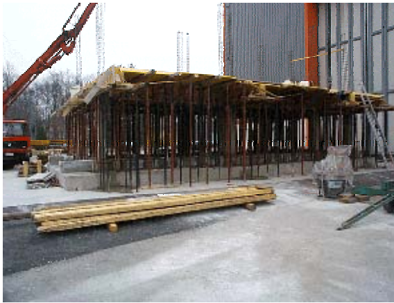
Figure A.7 - Casting of the 1 st floor (general view)
