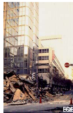
Figure 2.21 - Damages on buildings of different type in central Kobe (EQE, 1995)
