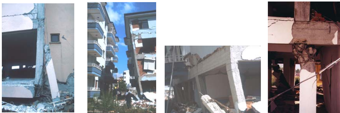
Figure 2.43 - Strong-beam weak-column mechanism (Aschheim, 2001; Saatcioglu et al. , 1999)
