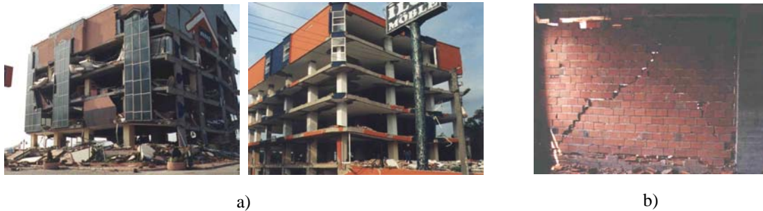
Figure 2.37 - Damages on masonry infill walls (Saatcioglu et al. , 1999): a) RC frame building with almost fully damaged masonry infills; b) diagonal tension failure of a masonry wall
