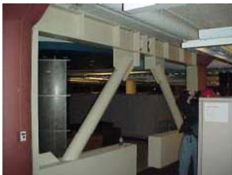
Figure 2.8 - Chevron eccentrically braced steel frame used to seismically upgrade building (Filiatrault et al. , 2001)
